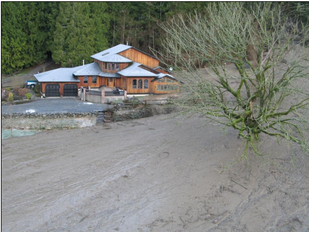
Figure 1 One of the homes affected by the debris flow on Chilliwack River Road, January 2009 (Gerraghty, 2009).
