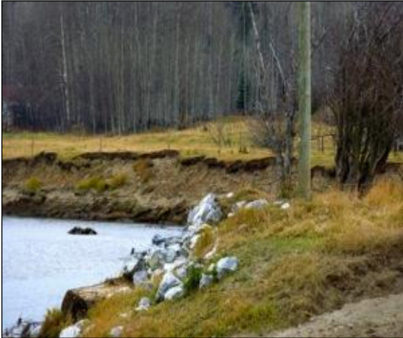
Figure 3. A photo of a riparian area at a ranch along the Chilako River near Prince George where a Livestock Watering BMP was installed. The bank lacks stability and in the years since installing the off-stream waterer and livestock exclusion fencing has been washed away during freshet events. This reach scored a 42.1% in a RHA (only a small portion is shown here). Examples such as this show that sometimes one BMP implemented in isolation will not achieve the environmental objectives it is meant to. This particular rancher indicated that peak flows and risks of flooding have increased due to the pine beetle management harvests in the area.
