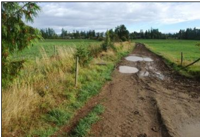
Figure 7. Example of a Riparian Buffer BMP along a constructed ditch that drains into a fish-bearing stream. The planted riparian vegetation is healthy; however, the riparian buffer was planned with only 1.5 m from the top of bank to edge of buffers. Two heavily used roadways flank each side of the buffer. This particular riparian area scored a 40%.
