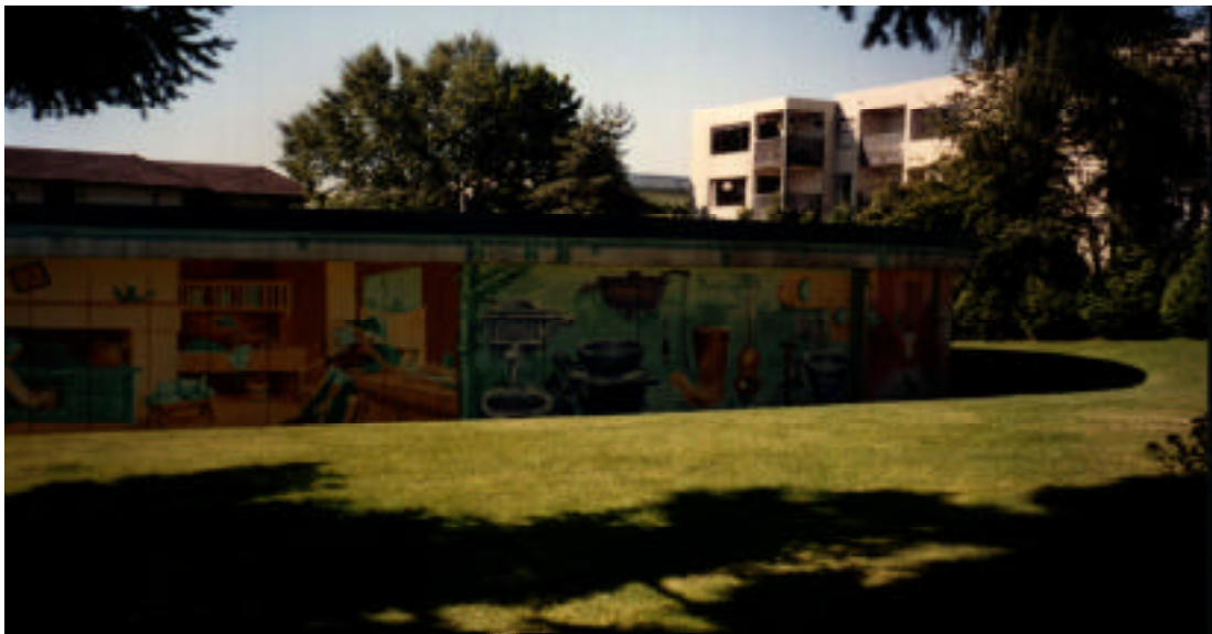
Figure 4.2 A concrete reservoir of the White Rock Utilities water system
