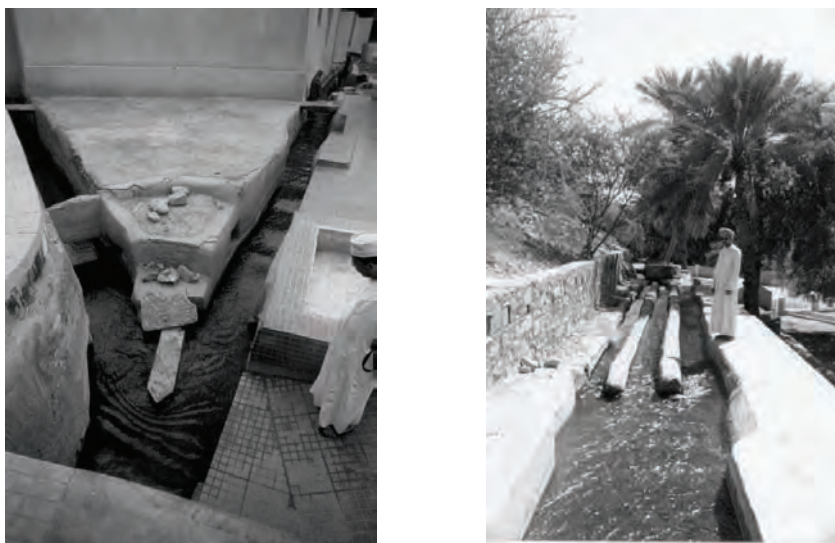
Figure 6. Flow division in aflaj systems.
