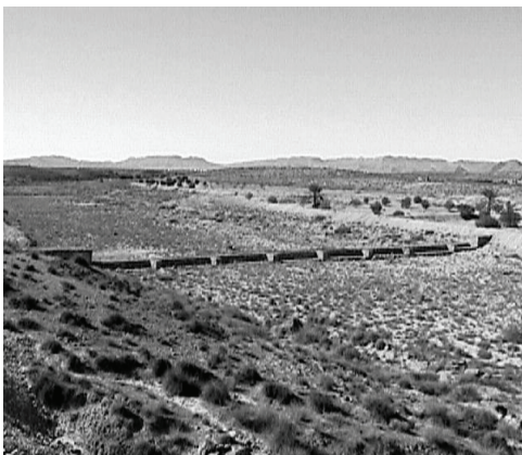
Figure 7. Gabion unit on Wadi Naguab .
